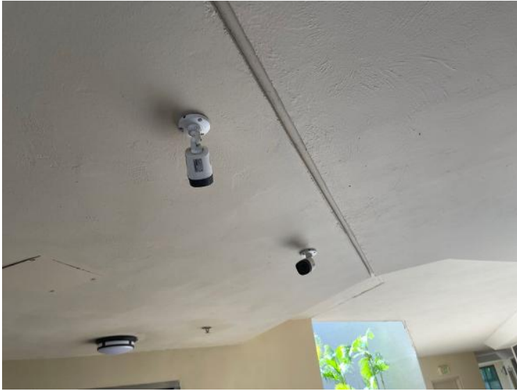
Photos / Fire Protections
