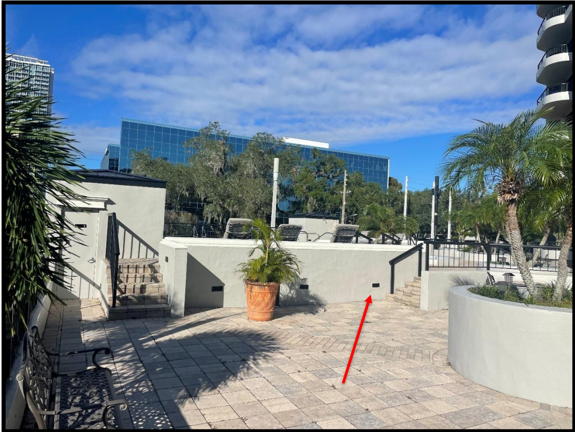
Overview of sun deck showing crawlspace ventilation
