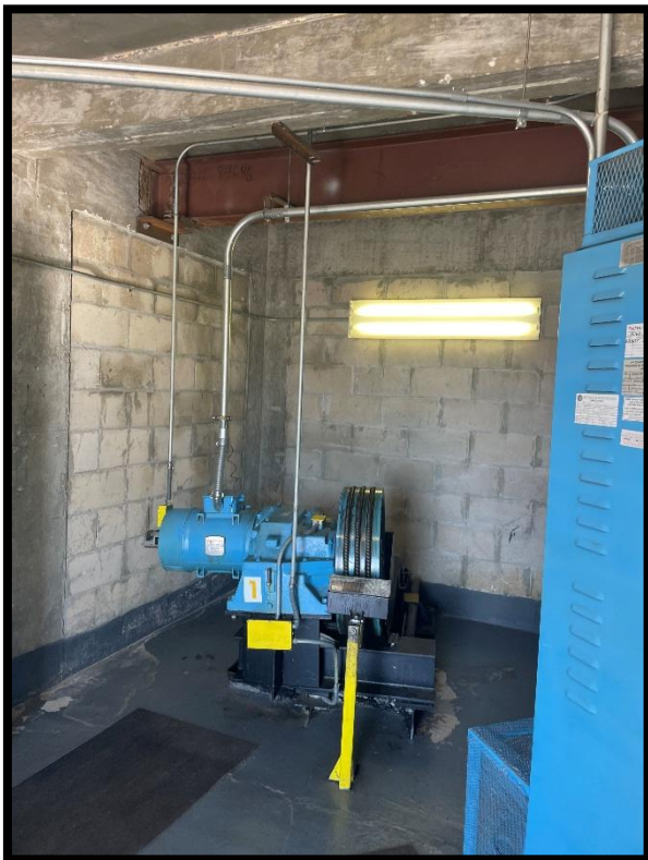
Elevator housing structure
