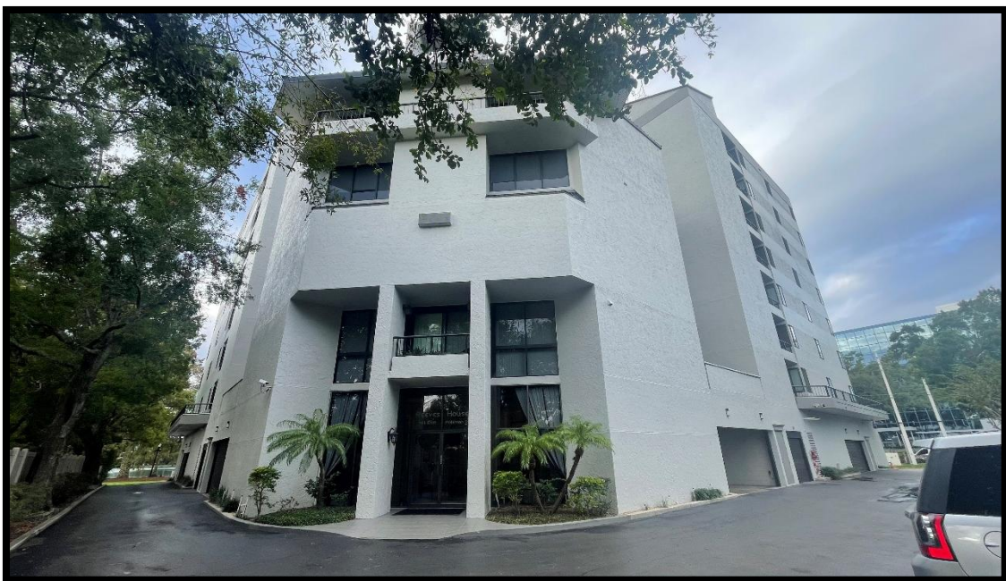
Northeast corner of the structure overview
