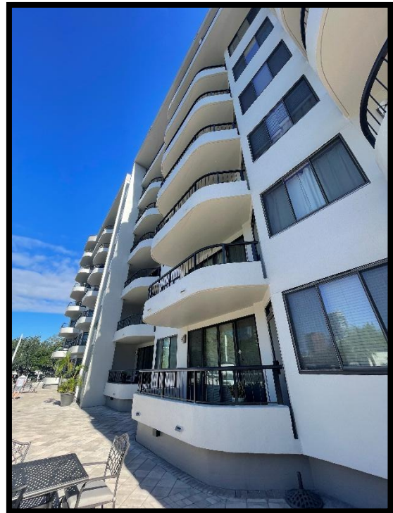
West corner of the structure overview
