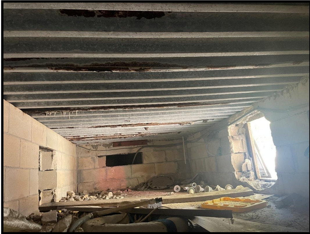
Metal pan bearing on CMU block stem wall
