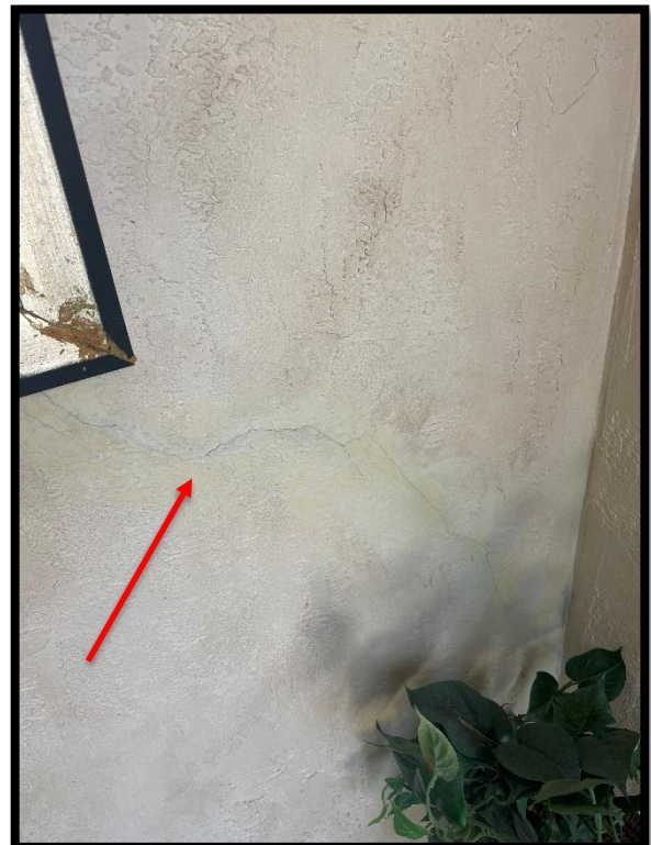
Repaired drywall crack in bathroom
