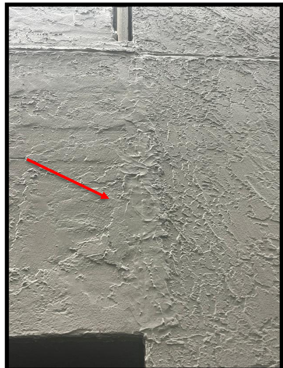
Recent touch-up on the stucco façade
