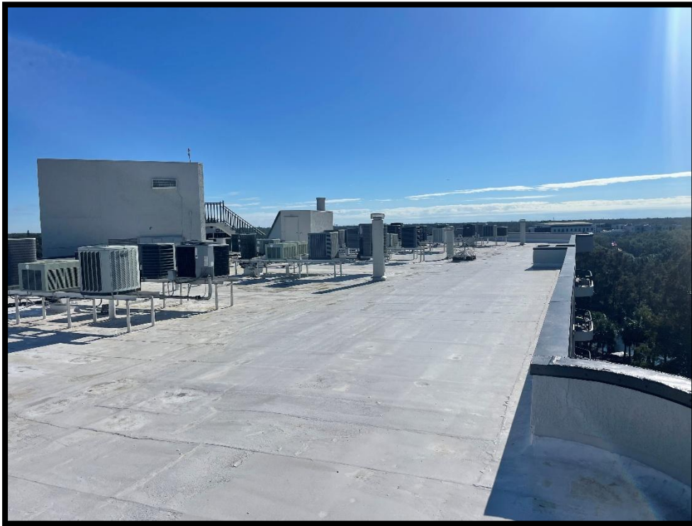
Overview of flat modified bitumen roof with parapet wall
