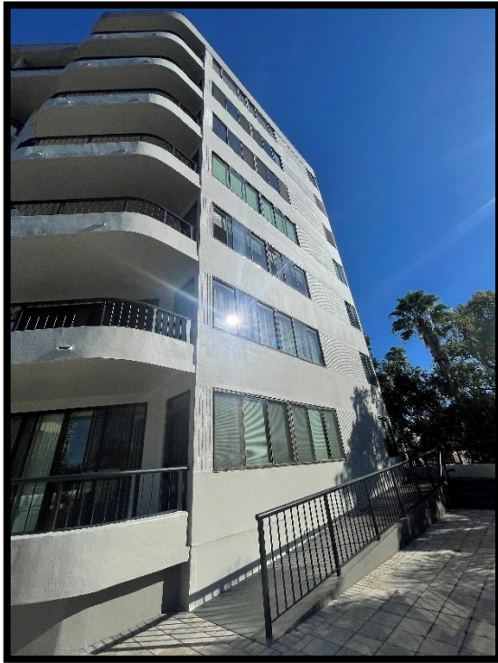
South corner of the structure overview
