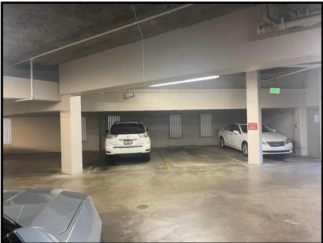
Beam deflection (performance) assessment
