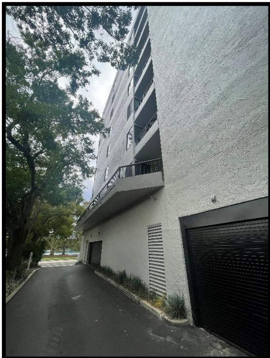
East corner of the structure overview
