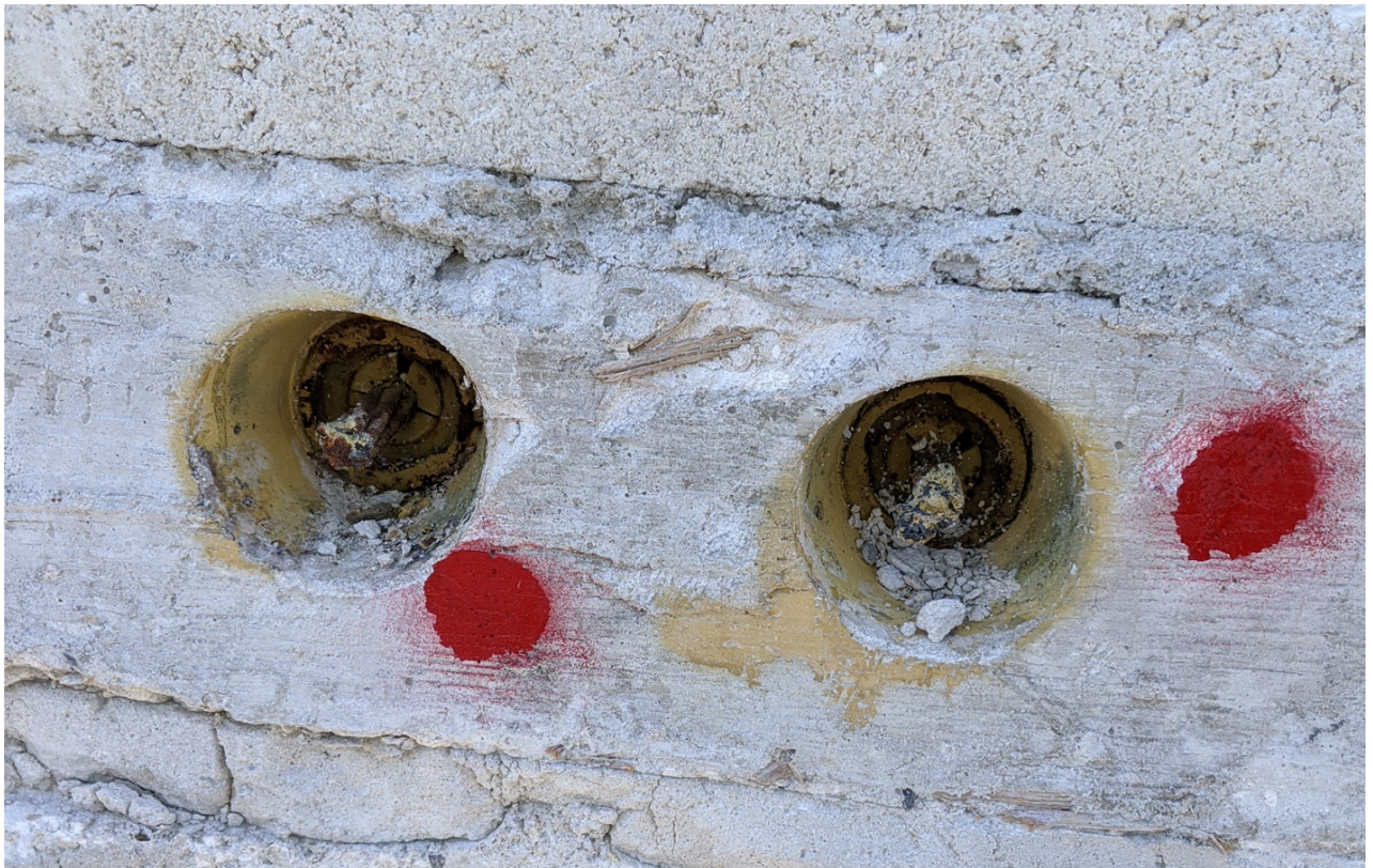
Picture of the typical tendon anchor corrosion of the slab edge. (Just an example from the same age building)
