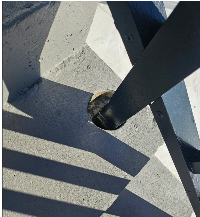
Picture of the typical post-pocket deterioration.
