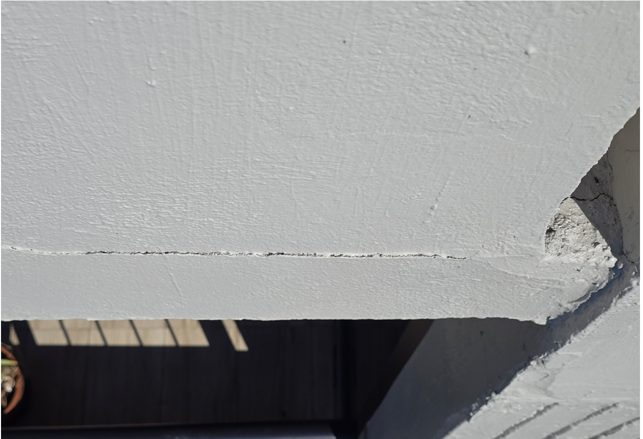
Picture of the balcony typical slab edge deterioration. PH level.
