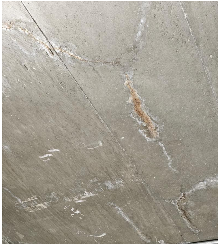
Picture of the elevator bulkhead roof slab with a visible crack underside of the concrete slab
