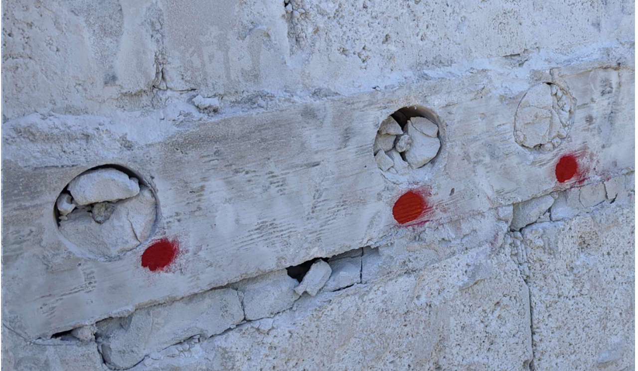
Picture of the typical PT pocket on the slab edge. (Just an example from the same age building)
